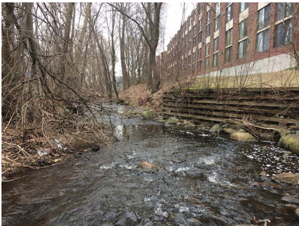
Photo 4. Erosion control “living wall” project along Mill Brook. (Private property)
