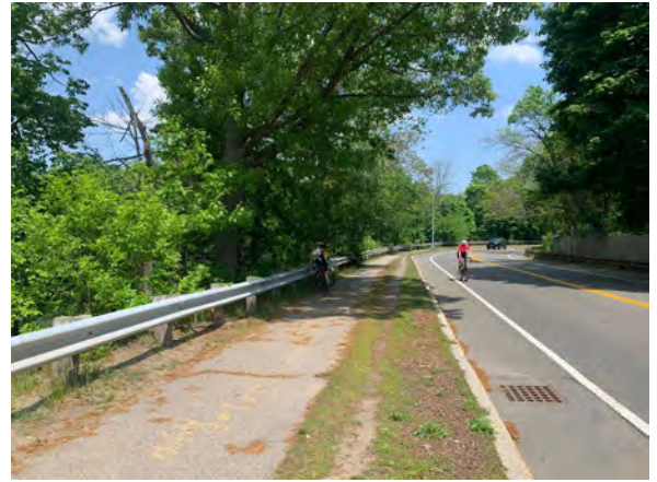
BEFORE: The existing path along the Mystic Valley Parkway is too narrow to support shared use, and only confident cyclists bike in the roadway.
