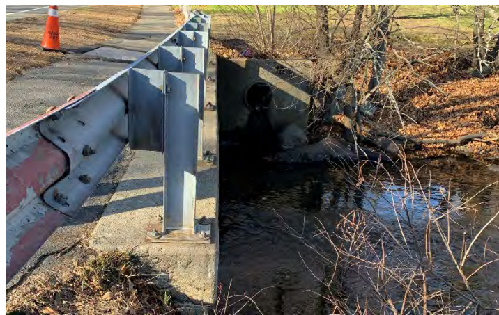
Figure 22 Concrete culvert over Mill Brook
