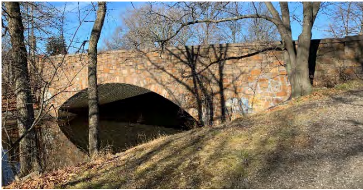
Figure 21 High Street bridge
