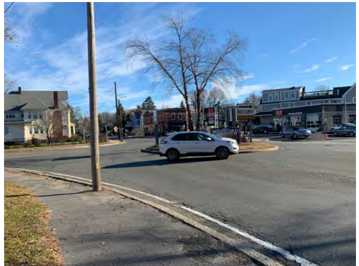
Figure 4: High Street rotary in Medford matches its Arlington counterpart in excess pavement, resulting in high vehicle speeds. This project proposes to establish safe walking and biking connections between the two rotaries and municipalities.
