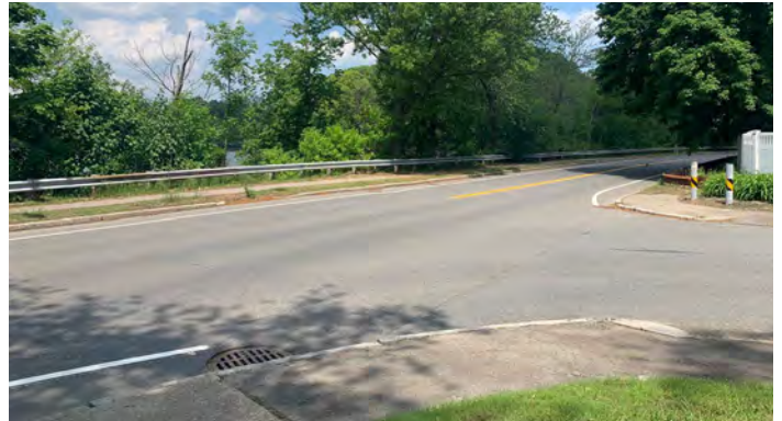
Figure 40: Mystic Valley Parkway at Hayes Street lacks a crossing
