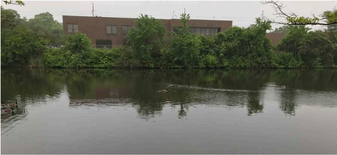
Inaccessible Riverfront with Dense Vegetation – National Grid
