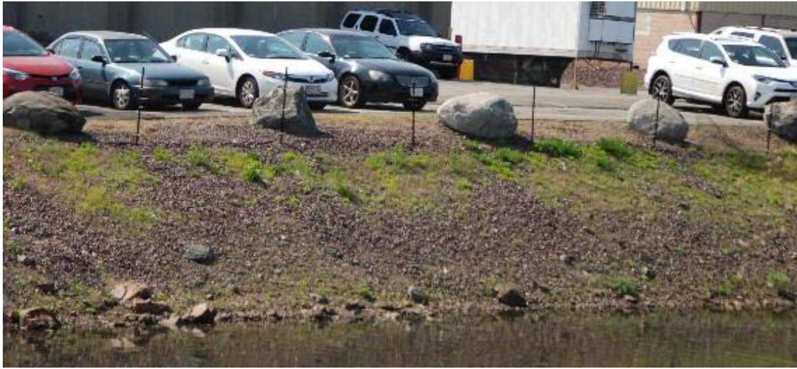
Inaccessible Riverfront with Parking at Edge – 240 Commercial Street (Piantedosi Baking Company)
