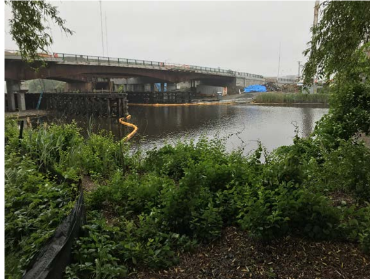
Revere Beach Pkwy reconstruction
