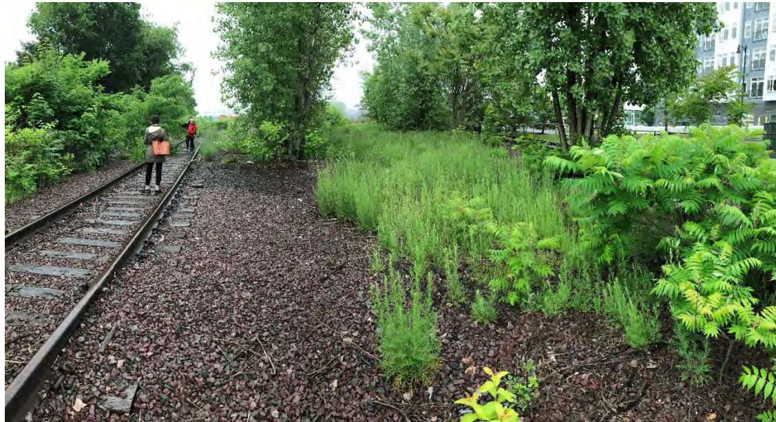
Rail line looking north at platform
