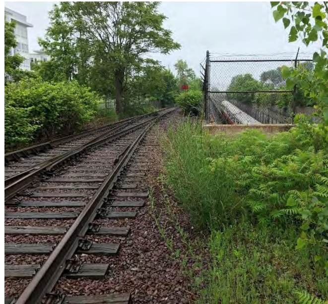
Rail spur capped over the MBTA line
