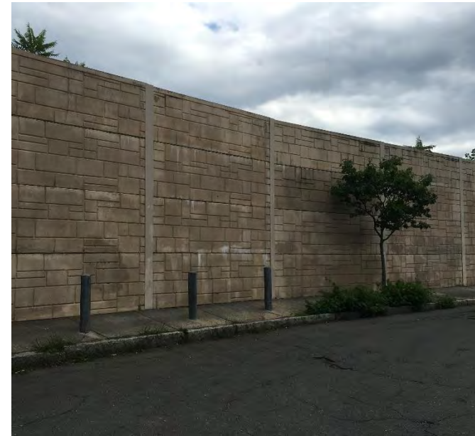
Sound wall and future access to rail park
